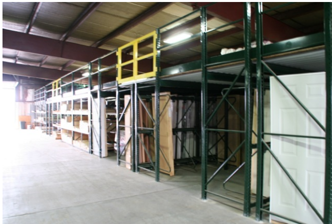
Mezzanine Storage in Bartlett's New Drive Thru
